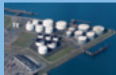
The Netherlands - Vopak Terminal Botlek (Noord)
