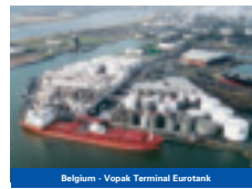
Belgium - Vopak Terminal Eurotank
