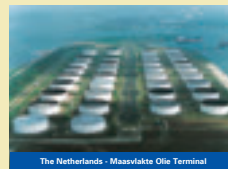
The Netherlands - Maasvlakte Oil Terminal
