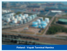
Finland - Vopak Terminal Hamina
