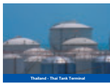
Thailand - Thai Tank Terminal
