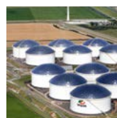
Page 205 Additional information Photo: Vopak Terminal Eemshaven (Netherlands)
