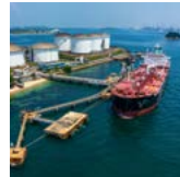
Page 112 Continuously challenging our systems and our processes Photo: Vopak Singapore - Sebarok Terminal (Singapore)
