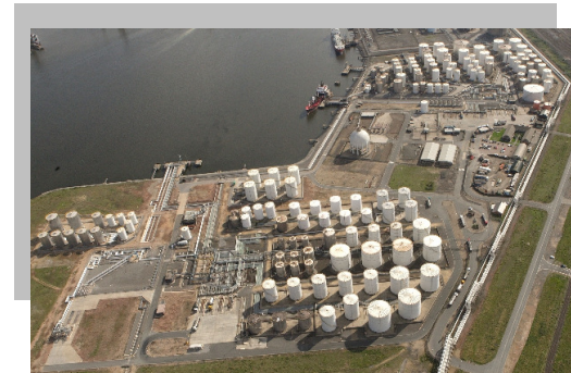
Teesside, UK Product: Chemicals Capacity: 40,000 cbm
