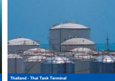
Thailand - Thai Tank Terminal
