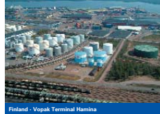
Finland - Vopak Terminal Hamina
