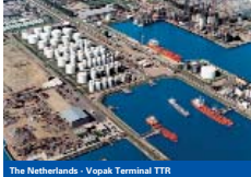
The Netherlands - Vopak Terminal TTR
