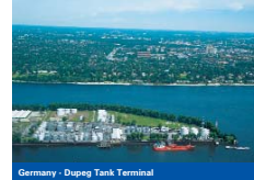
Germany - Dupeck Tank Terminal
