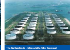
The Netherlands - Maasvlakte Olie Terminal
